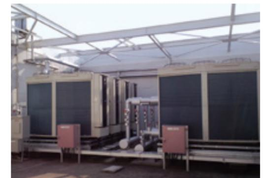
Introduction of highly efficient hot/cold water heat pump chiller (Ube Plant)
